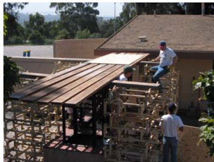
Here they are setting up the platform to hold the roof.
